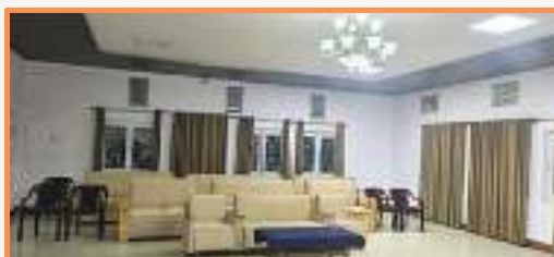
Renovation of School Ante Room.
