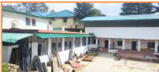
Renovation of existing BVN building for Girls' Hostel.
