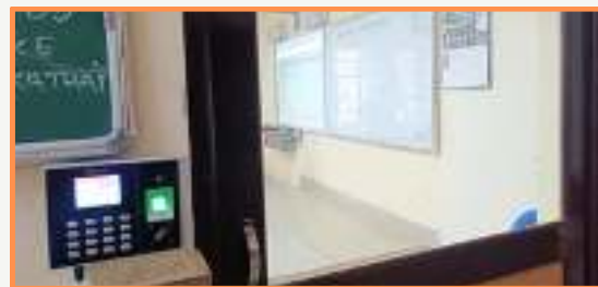
Installation of RFID system in the classrooms.
